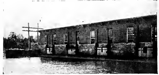
FIG. 9.—EXTERIOR OF POWER HOUSE, CONCORD, N. H., WATER POWER PLANT.
